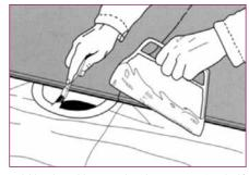
Fold back and loosen the sheets covering half of the floor area. Apply the adhesive on the subfloor with a fine-notched trowel. Use a soft brush around drains and hard-to-reach areas. Around and inside drains, please see drain manufacturers recommendation.
